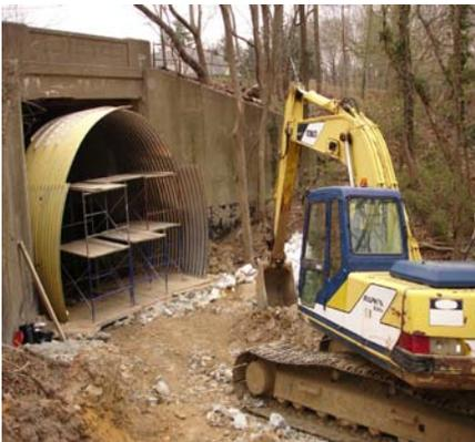
*Excavation and Insertion of Steel Arch— Later a Concrete Arch will be Poured*
